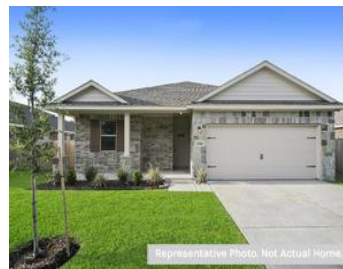
11033 Patriot Court Cleveland, TX 77328
