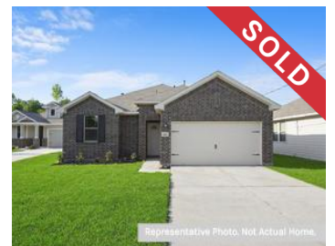
11044 Patriot Court Cleveland, TX 77328
