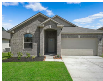
11041 Patriot Court Cleveland, TX 77328
