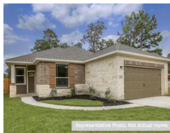
11037 Patriot Court Cleveland, TX 77328
