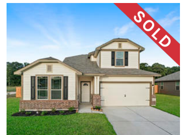
11005 Patriot Court Cleveland, TX 77328
