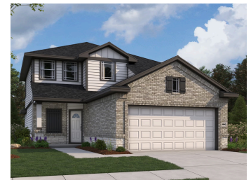
2965 Buckthorn Drive Brookshire, TX 77423
