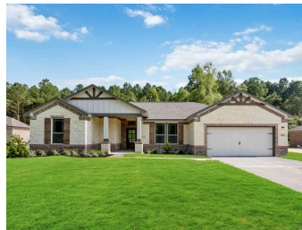
1538 Vista View Drive Pleasanton, TX 78064
