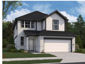
2314 Dry Moss Way San Antonio, TX 78224
